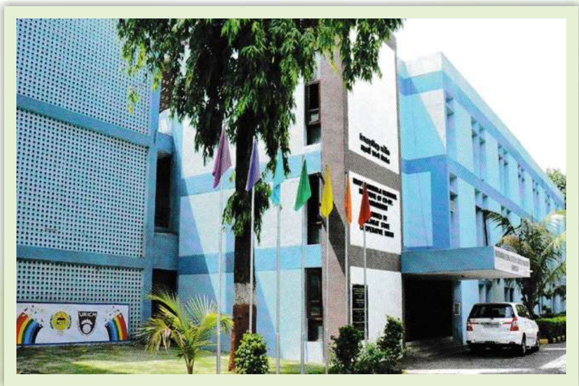
Administrative Block of URICM, Gandhinagar
