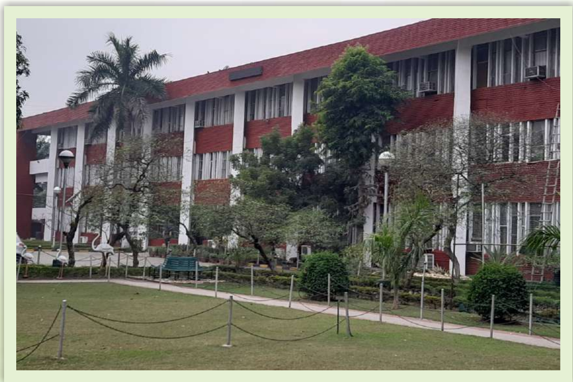
Administrative Block, RICM, Chandigarh
